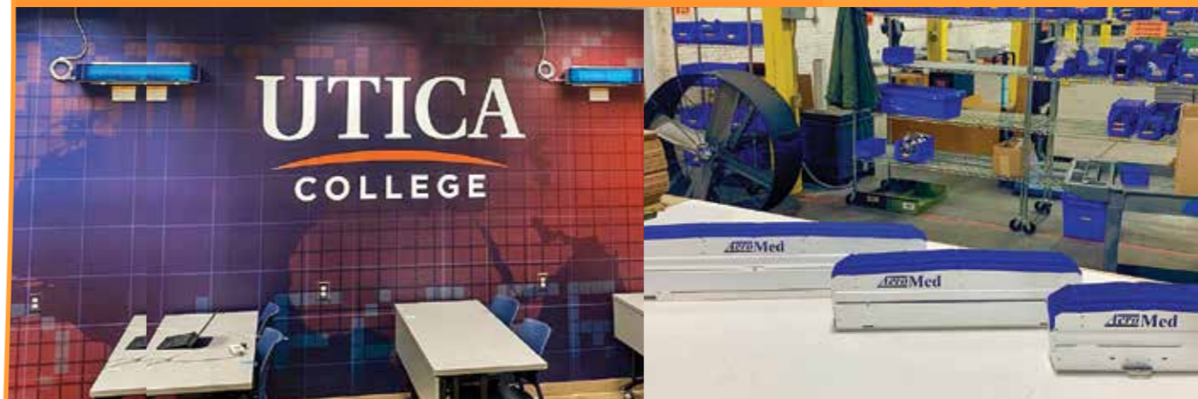
Upper room UV disinfection units in action at Utica College
